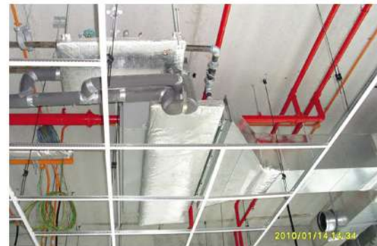
Ducted Fan Coil Unit
