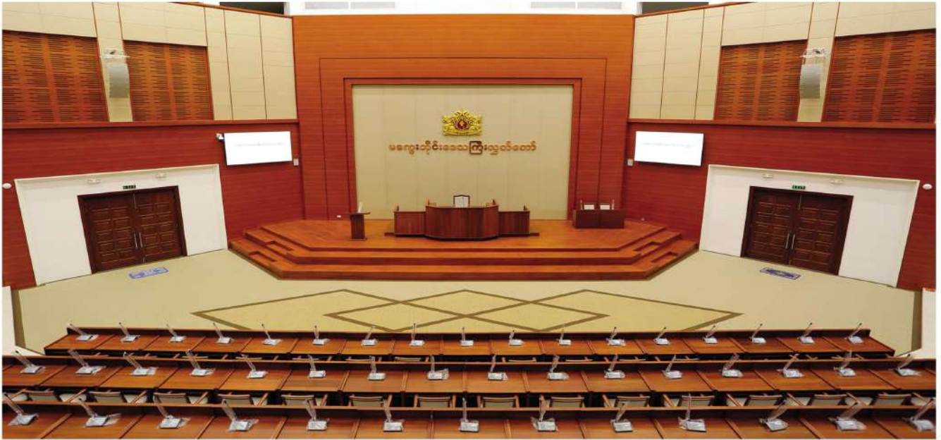
Public Address & Conference Voice Control System
