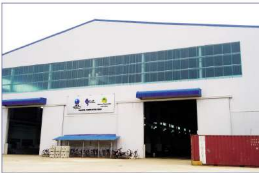
J&M Steel Fabrication Factory
