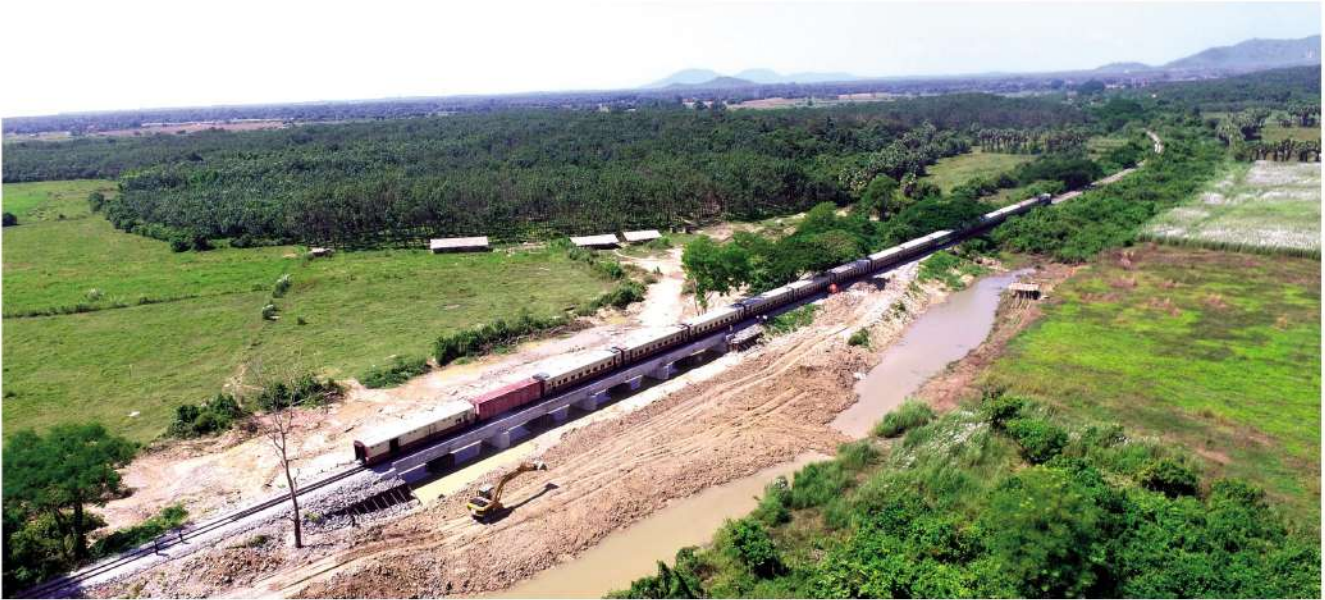
Bridge No. 72(A) Project
