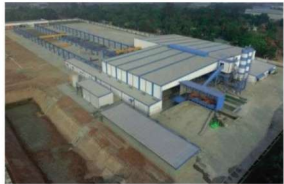
I&H Engineering Precast Concrete Factory (Hmaw-Bi)
