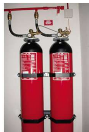
Gas Suppression System
