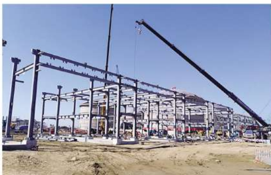
Truck Loading Bay (TLB), PSW Terminal Project
