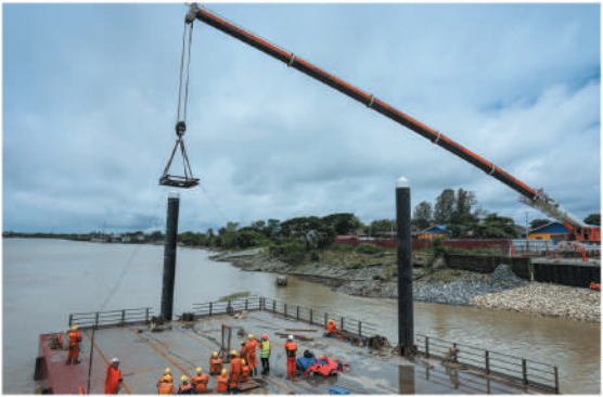
Pile Guide Installation
