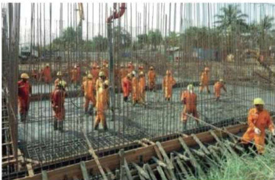
Concreting Work (Water Tank)
