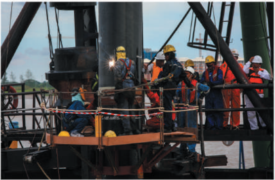
Pile Splicing
