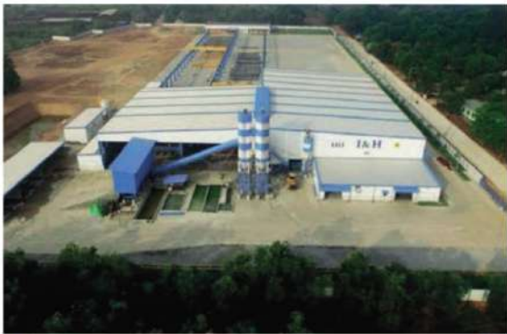
I&H Engineering Precast Concrete Factory (Hmaw-Bi)
