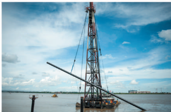
Pile Driving by Piling Barge
