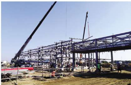
Pipe Bridge, PSW Terminal Project
