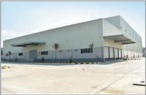
Automated Warehouse for Pharmaceutical Factory
