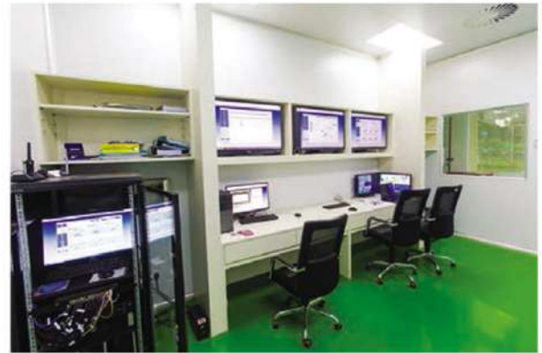
Building Monitoring Station
